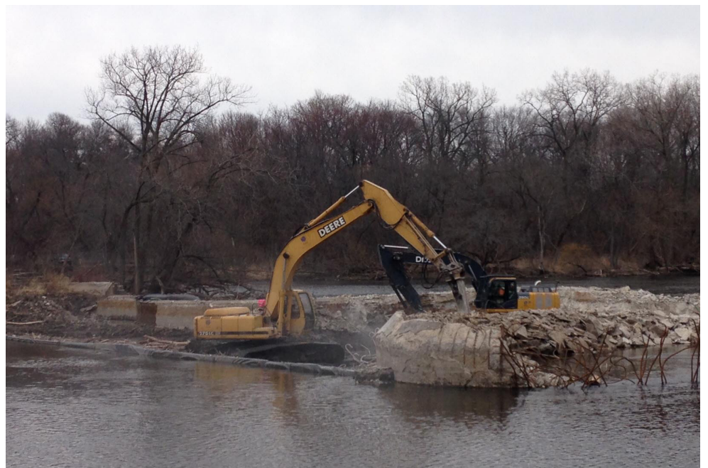
Removal of Estabrook Dam
