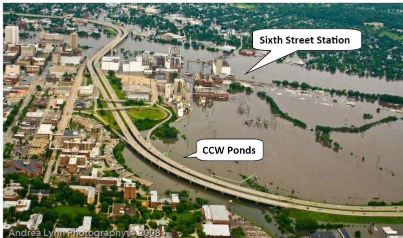
Figure 1. Sixth Street Station at Flood Peak, June 13, 2008. 144
