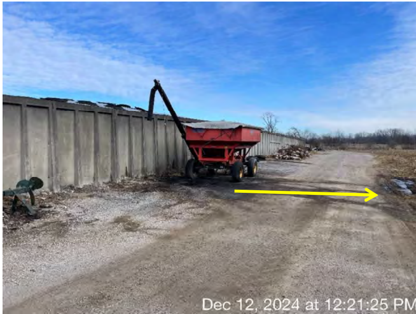
Photo 22. An area where leachate seeped through the southern bunker wall. Leachate flowed south across the adjacent driveway and entered the field located south of Site 1.
