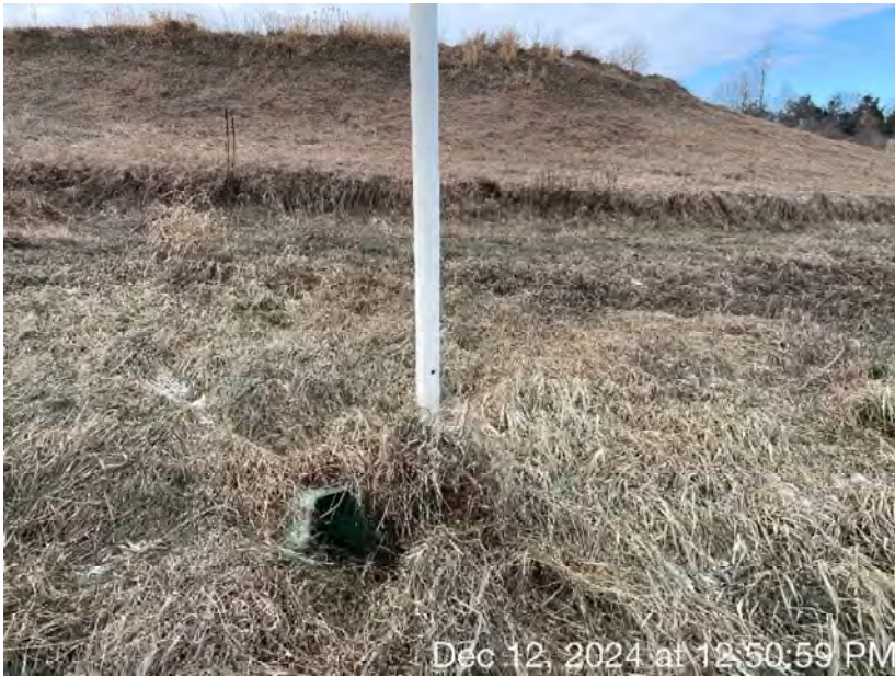
Photo 36. A culvert that diverts stormwater from the production site at Site 2. This outlet is located east of the outdoor concrete lot.
